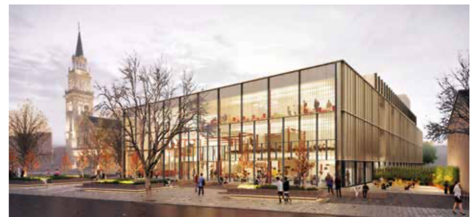
Work has progressed on our new Student Centre, including a new Students' Union facility
