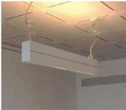
Figure 3. Luminaire with direct and indirect light output.
