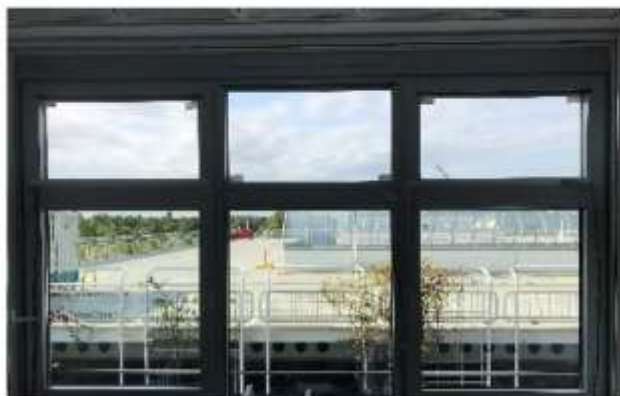
Figure 2. The façade seen from the inside, with the light-emitting structure on the upper part of the window.
