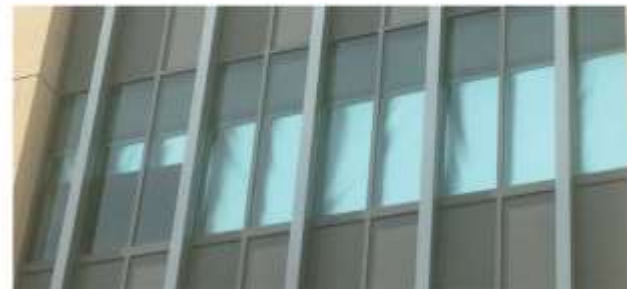
Figure 8. Outdoor view of the upper blinds (dark grey) and lower reflective shades (white) with the lefthand lower shade partially raised, coming out of the bottom and sides of the DZSC shades. During cool or cold weather, temperature conditions were deemed "just right".
