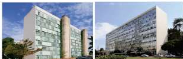
Figure 2. West and East façades of the building.
