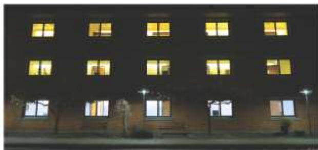
Figure 2. Exterior night view of Vikaergaarden rehabilitation facility with existing fluorescent lighting (two top floors) and new dynamic LED lighting (bottom floor).
