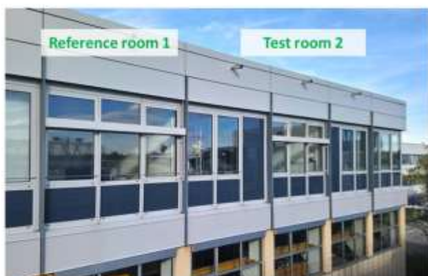
Figure 4. An exterior view of the lab. The façades of both the reference and test room can be seen in the picture.
