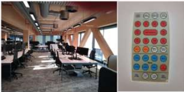
Figure 2. (Left) Inside the open plan office at Aurecon Brisbane. (Right) Hand-held remote presence sensor controller (Servodan 41-926) to override automated dimming or turn luminaires on-off.
