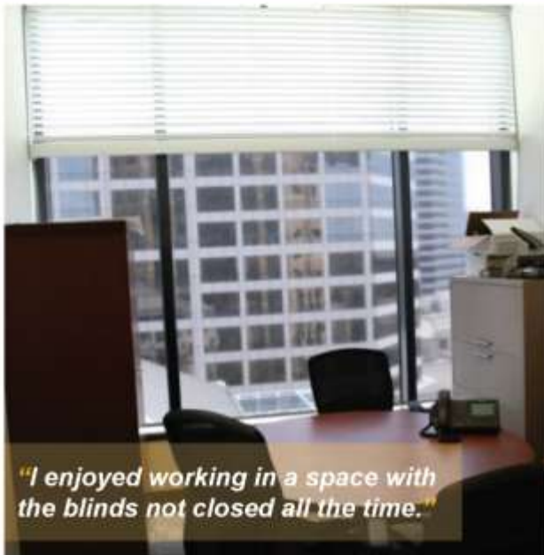
Figure 7. Indoor view of the DZSC GG tinted shade when fully lowered. ride was provided with automation of the upper blind, but control of the blinds was grouped to lower the cost of installation, so comfort control per individual preferences was constrained even in the private offices.
