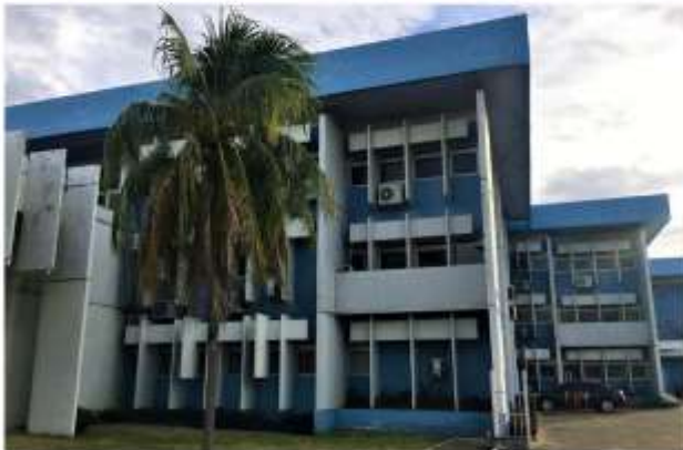
Figure 2. Forum Sobral Pinto, Northeast Façade.
