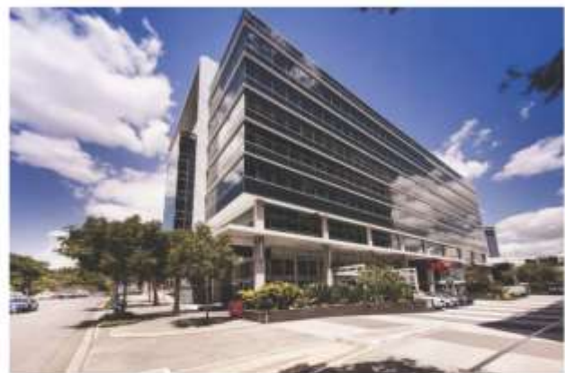
Figure 1. AECOM Brisbane's open plan office located in Brisbane, Australia.
