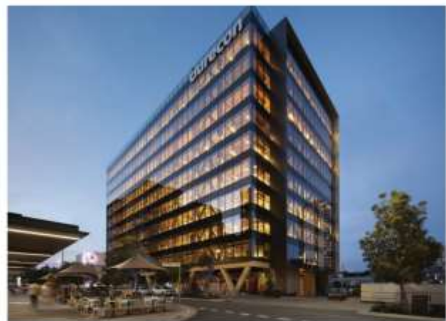
Figure 1. Aurecon's open plan office located in Brisbane, Australia. Image sourced from: https://www.archdaily.com/906495/the-tallest-timber-tower-in-australia-opens-in-brisbane
