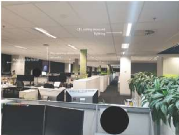
Figure 2. Photo inside AECOM Brisbane showing a portion of the open plan office where occupancy sensors, CFL lighting and manual blind shades are used as part of their lighting system.
