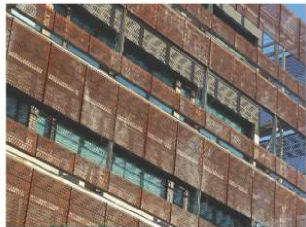
Figure 1. South view of the double skin microperforated façade of IDOM Headquarter in Madrid. This façade is perhaps its most distinctive sign. The façade, which was designed to reduce overheating, provides also some glare protection if combined with roller shades.
