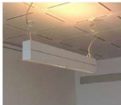
Figure 3. Luminaire with direct and indirect light output.
