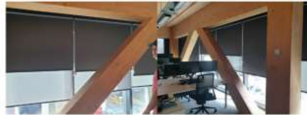
Figure 11. Real outcomes from conducting a POE survey, where glare was reported by a significant number of occupants. Additional blinds were installed with lower VLT (<10%), to deliver a double roller strategy for increase control of daylighting.
