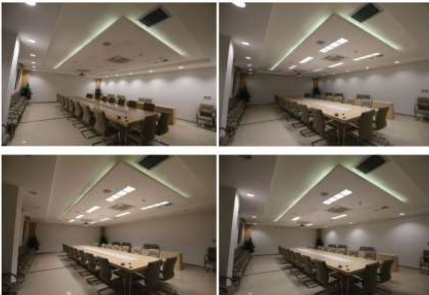
Figure 9. Lighting environment for different scene settings (or "modes") in the video conference room equipped with LED.
