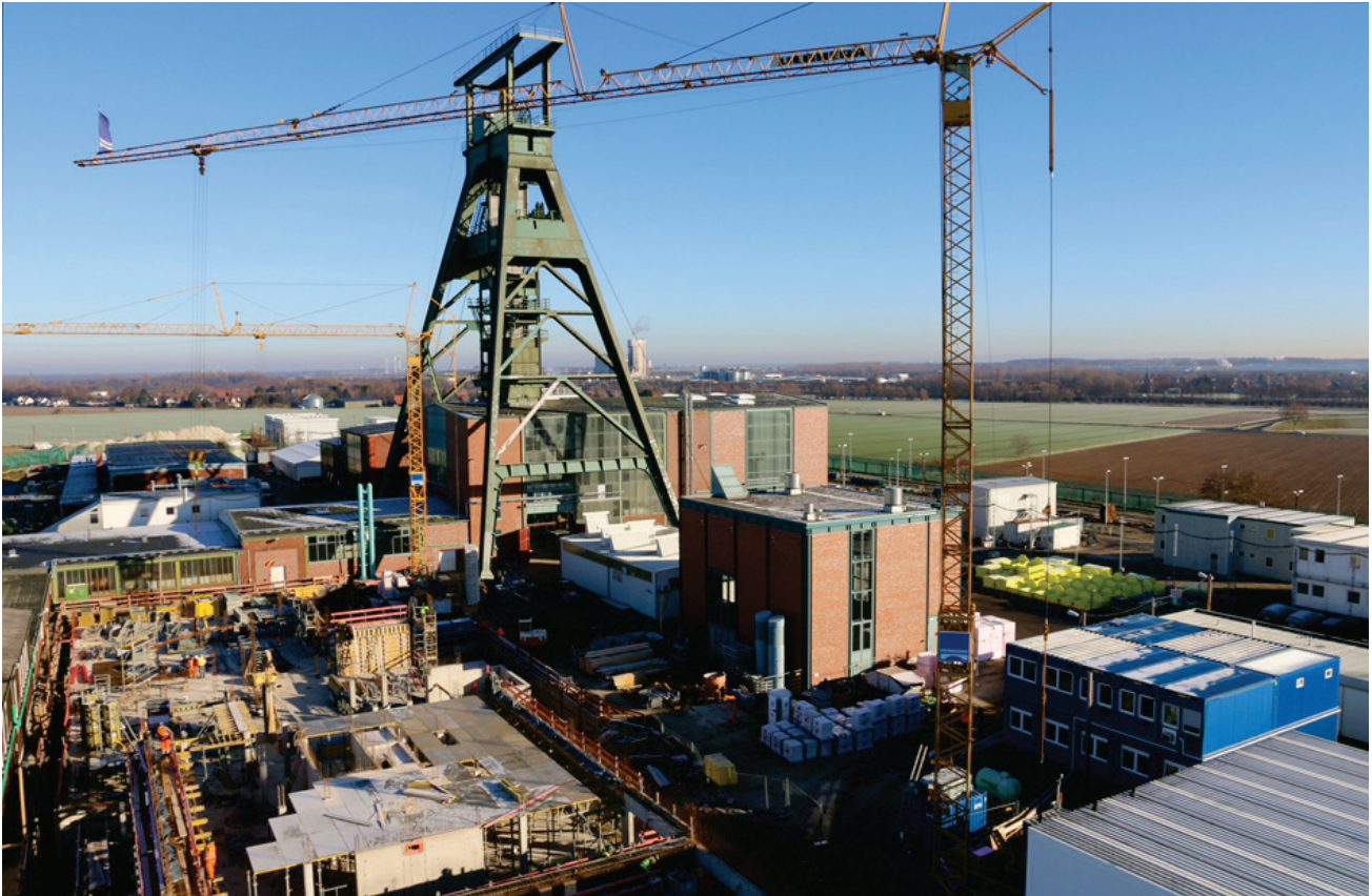
Figure D-10: Konrad repository construction site in Salzgitter (Copyright: BGE)
