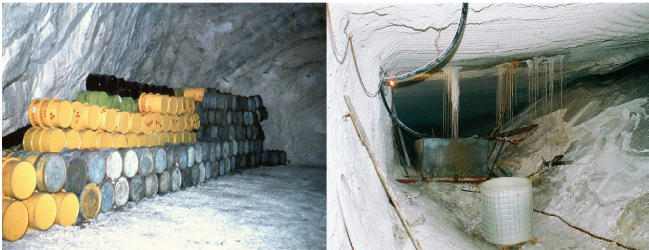
Figure D-11: Asse II mine (left: waste packages in an emplacement chamber (no more accessible today), right: dripping point) (Copyright: BfS)
