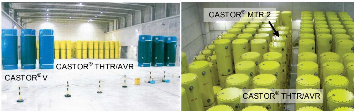
Figure D-5: Transport cask storage facility Ahaus (Copyright: GNS) left: CASTOR ® V and CASTOR ® THTR/AVR right: CASTOR ® MTR 2 between CASTOR ® THTR/AVR
