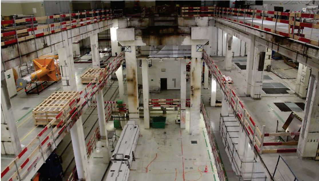
Figure D-15: View into the empty turbine building of the KWO (Copyright: EnBW)
