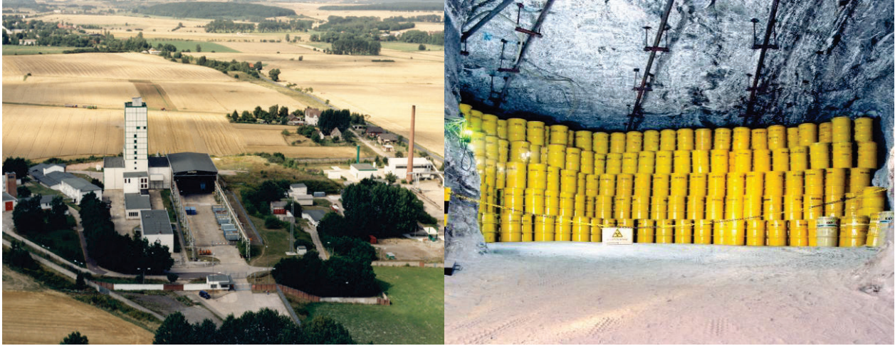
Figure D-9: Morsleben repository for radioactive waste (ERAM) (left: aerial view, right: emplacement chamber with stacked low level waste drums) (Copyright: BfS)
