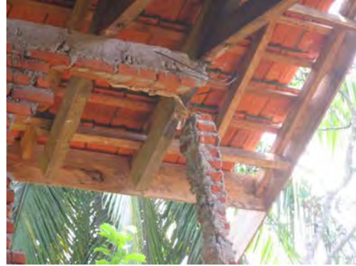
Figure 17. Confined masonry house with failure in masonry walls and connections between tie columns and bond beams, Kec. Airnapal (North Bengkulu)
