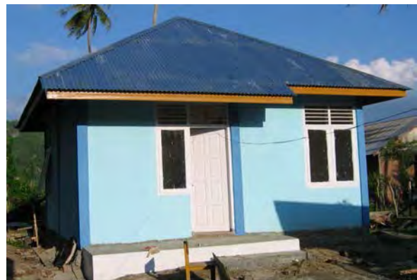
Figure 10. Rabung Empat Roof (Rusdi Razali's house designed and built by Build Change, Keunue ue, Peukan Bada, Aceh Besar)
