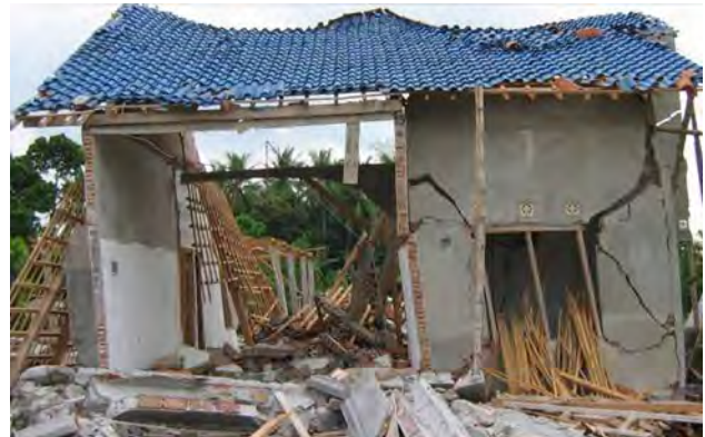
Fig. 3. Confined masonry house under construction, insufficient connections, Pleret (Bantul). S7.87574°, E110.40703°, IMG_6575
