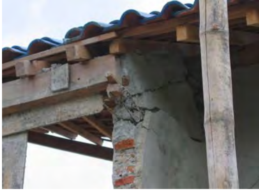
Figure 16. Zoomed in view of ring beam column connection. IMG_6577
