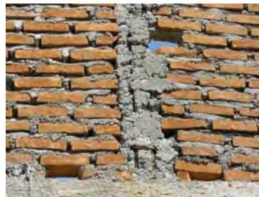
Figure 16. Typical wall built by Build Change-trained mason
