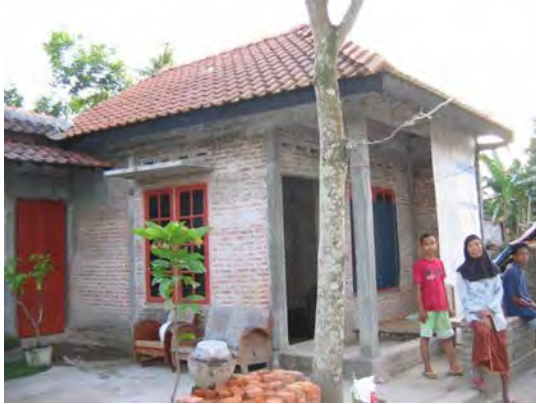
Figure 1. Well designed and built confined brick masonry house, edge of heavily damaged Pleret (Bantul), S7.83686° E110.41552°, IMG_6636
