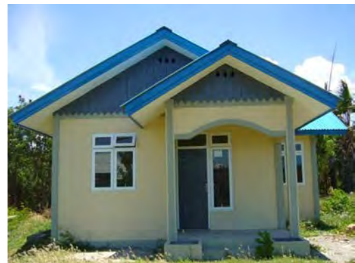
Figure 15. Covered terrace with lightweight wall, Build Change designed house for Catholic Relief Services (Aceh Besar)
