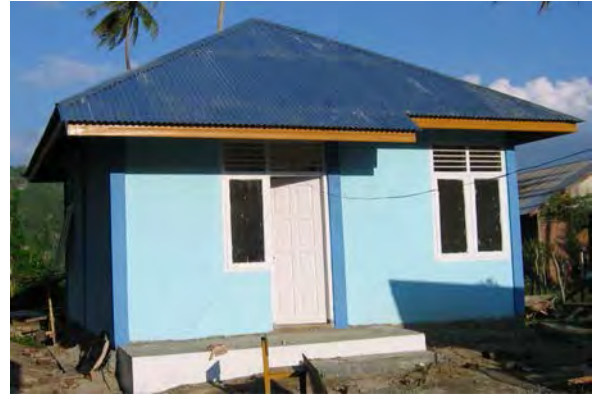
Figure 7. Rabung Empat Roof (Rusdi Razali's house designed and built by Build Change, Keunue ue, Peukan Bada, Aceh Besar)
