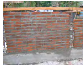
Figure 17. Typical wall built by Build Change-trained mason
