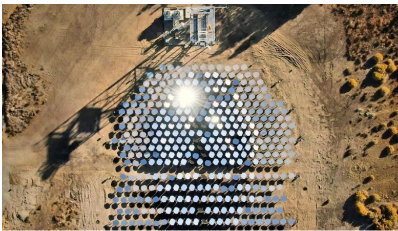
An advanced solar thermal plant built in Lancaster, California, has successfully reached the very high temperatures needed for many industrial processes. Photo source: Heliogen
