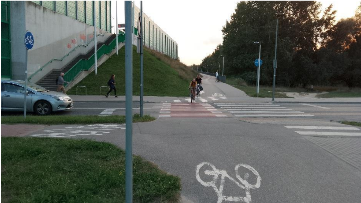
Figure 3. Świderska Street, Warsaw, Poland. The cycle ramp leading from a bridge ends on a crossing with a local road without good visibility splay and without clear priority established. Six car-cycle accidents have been registered on the crossing between 2014 and 2022.
