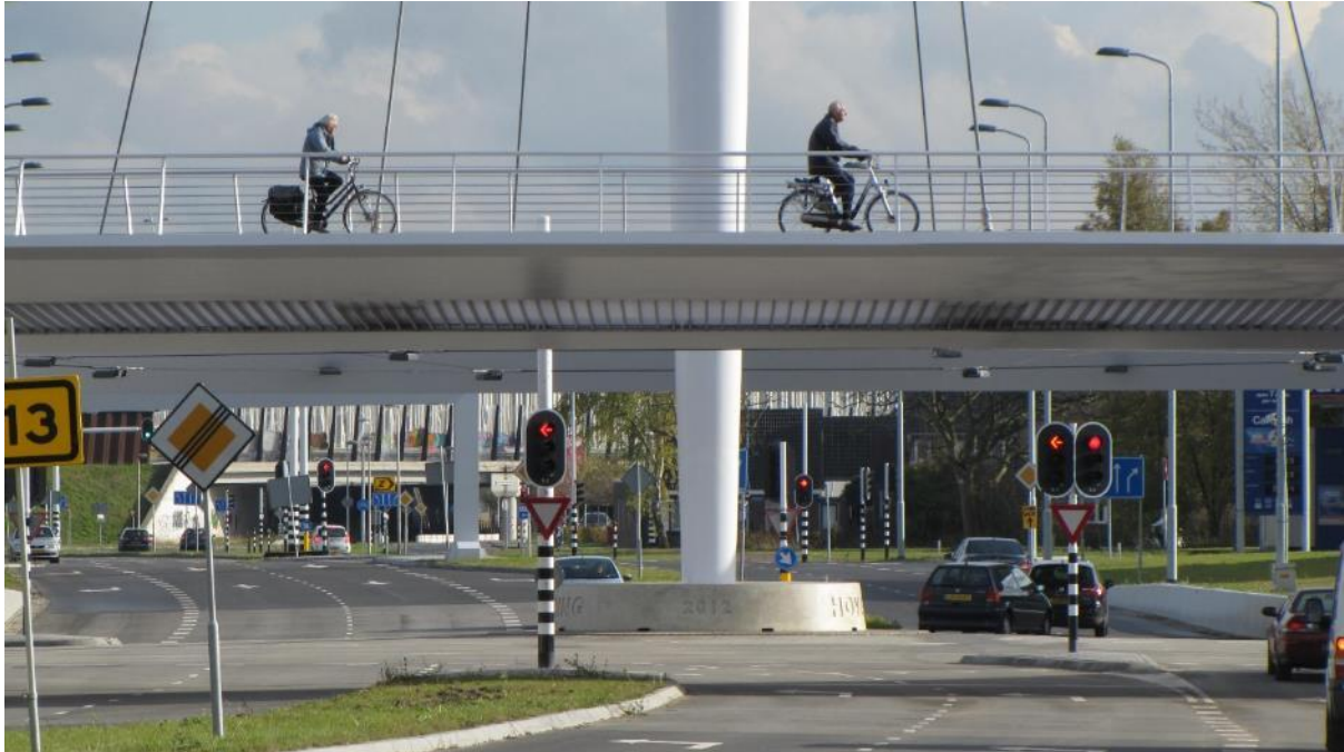
Figure 6. The Hovenring cycle bridge over a major road intersection near Eindhoven, Netherlands. To reduce the elevation change for cyclists, the intersection of carriageways was lowered by 1.5 m. As a result, the ramps leading to the bridge have gentle gradients between 1.86% and 3.09%
