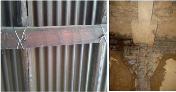
Fig. 24. Showing GI wires, threaded rods and metal plates used in the construction
