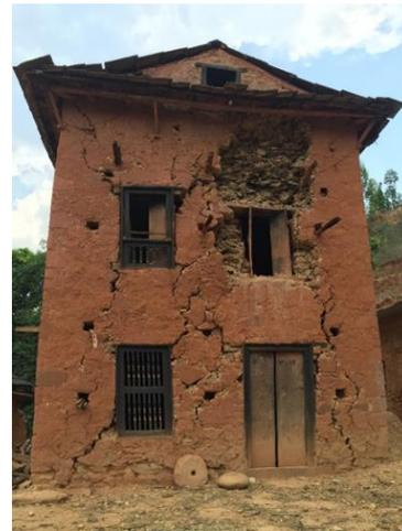
Fig. 9. Short wall damage
