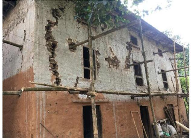
Fig. 26. Damaged house prior to retrofitting
