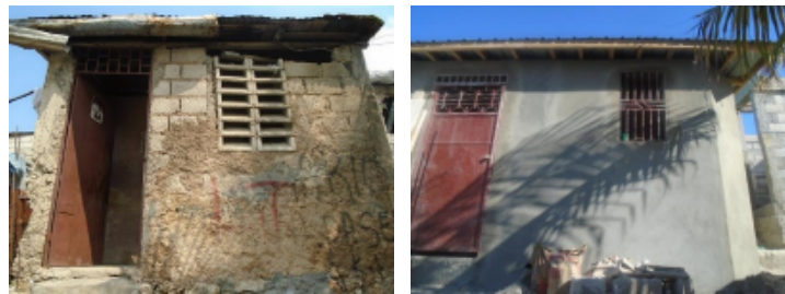
Fig. 4: A home in Port-au-Prince before (left) and after (right) a seismic retrofit
