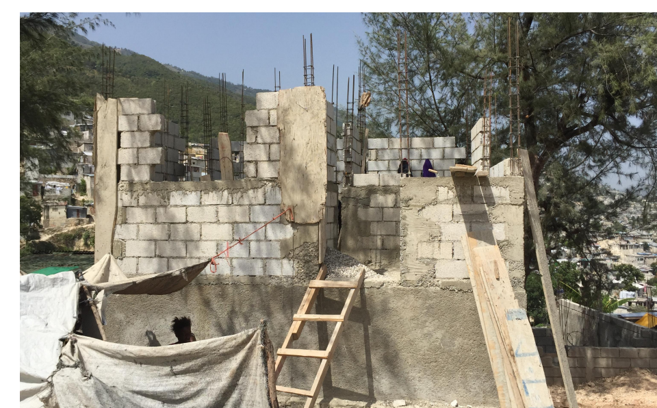
Confined Concrete Block Masonry (low ductility)
