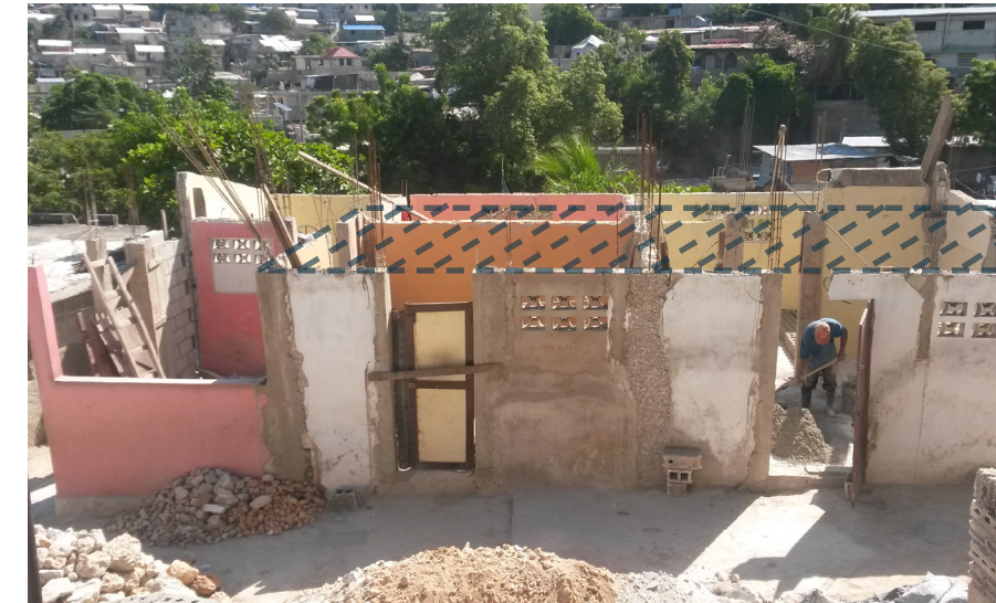
1. Destroy the lightweight roof or the damaged concrete roof.
