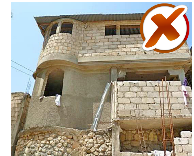
The geometry of the expansion should be regular and respect the geometry of the lower floor plan.
