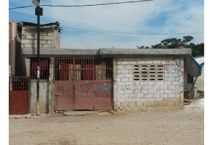
Unreinforced masonry house
