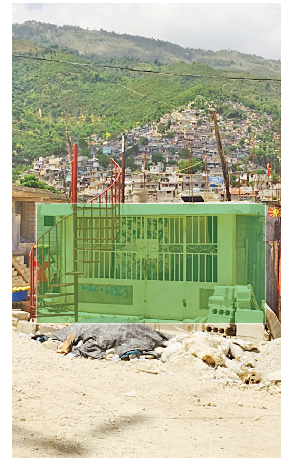
1- Retrofit existing building
