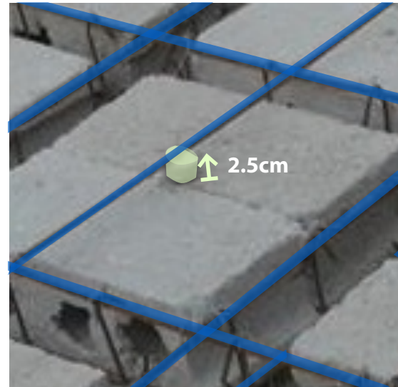
13. Use spacers to maintain 2.5cm of covering on the block. (Cf. Retrofit Practical Handbook 1 , "Concrete Spacers" page 5).
