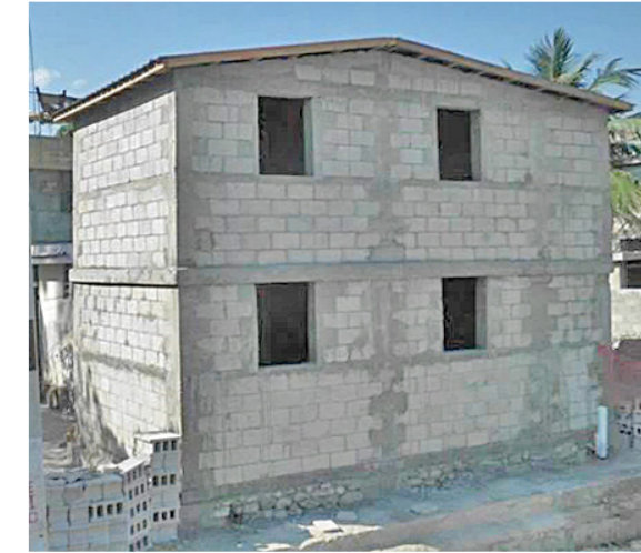
Confined masonry house
