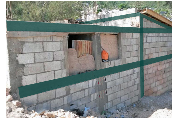
Lightweight roof with a second story wall
