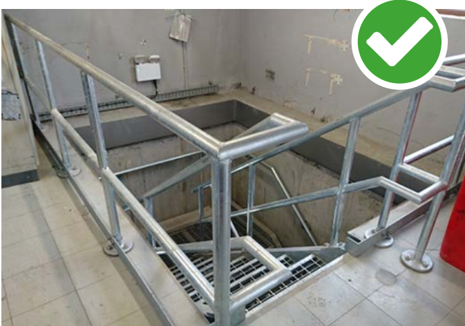
Image 5.2 Safe and easily accessible stairway to confined space
